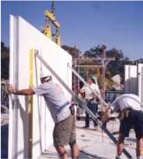
Panel being propped
