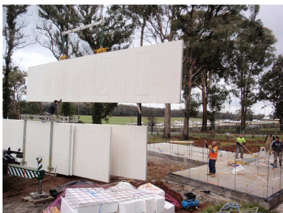
Panel being removed from stillage
