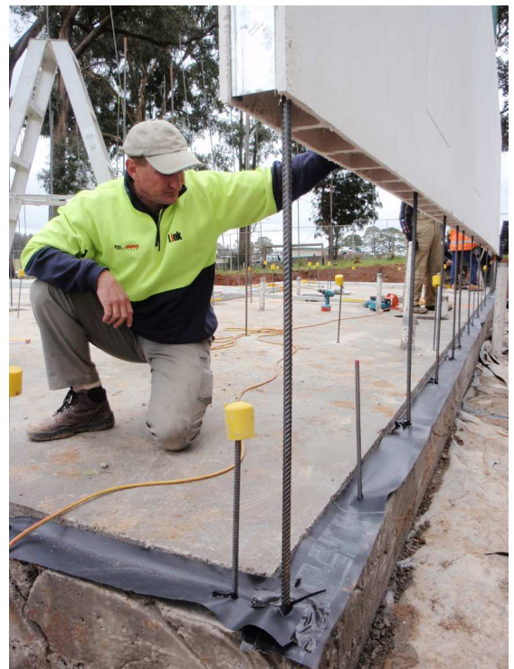
Lowering panel into position over starter bars and waterproof membrane
