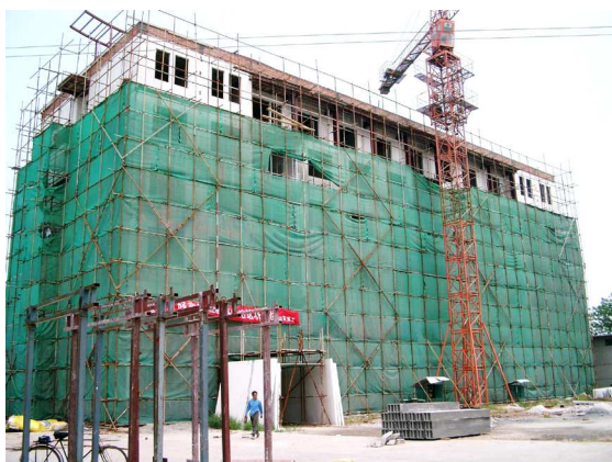
Multi-storey building using tower crane
