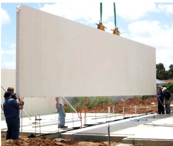
Double lifting jaw lift of large panel
