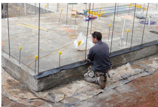
Prepare slab for panel installation
