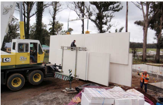
Removing panel from stillage
