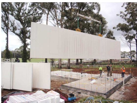
Panel being lifted into position
