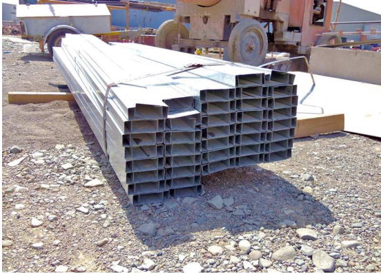
Metal studs: 92mm x 135mm x 1.15 bmt
