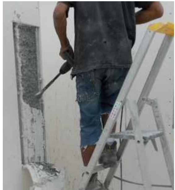
Repairing a concrete blowout
