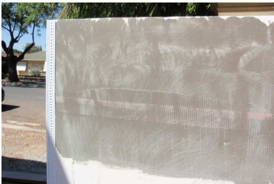
Section of joined panels showing fibreglass tape and corner bead
