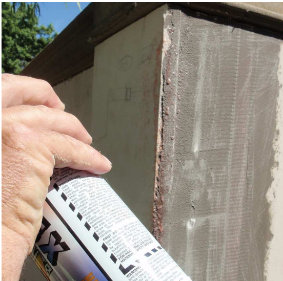
Applying trim spray adhesive prior to installing corner bead
