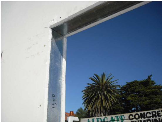
Vertical and Horizontal metal studs fitted in opening
