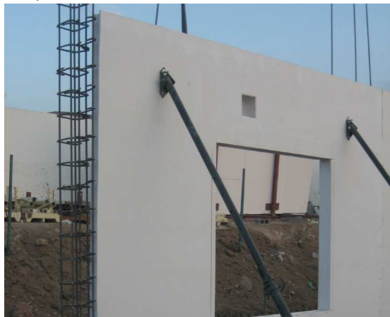
Top of prop with pivoting bracket
