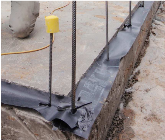
Reinforcement bars and damp proof course installed
