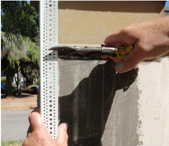
Cutting external corner bead to size
