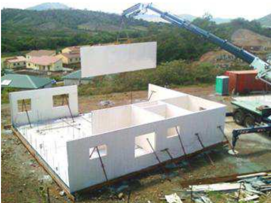
Craning panel into position.
