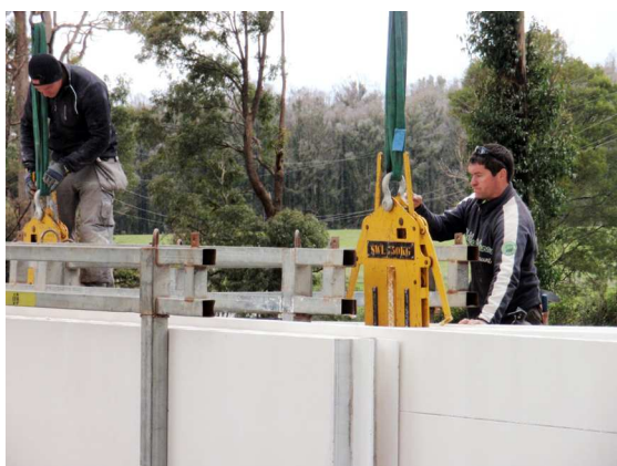
Lifting jaws being lowered into position
