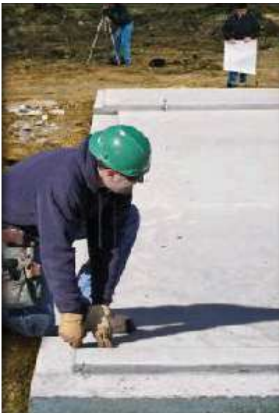
Checking the accuracy of the slab
