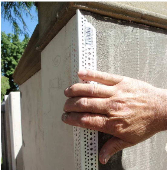
Affixing corner bead after application of trim spray adhesive
