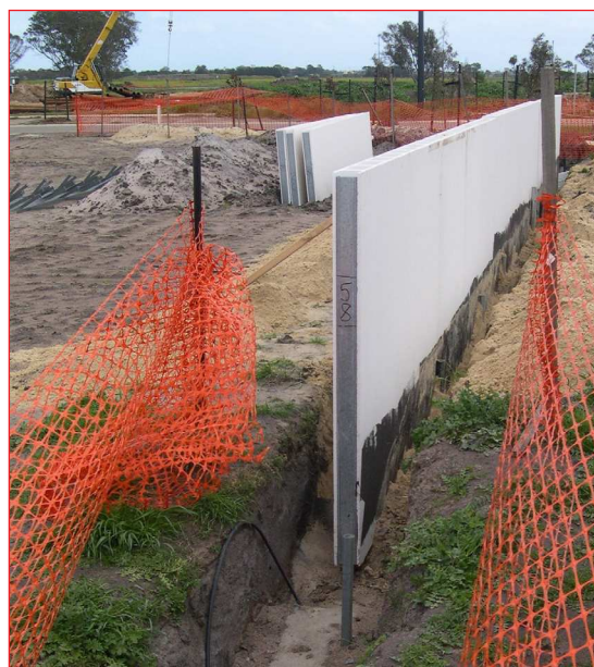
Rapidwall fence preparation for filling with sand.
