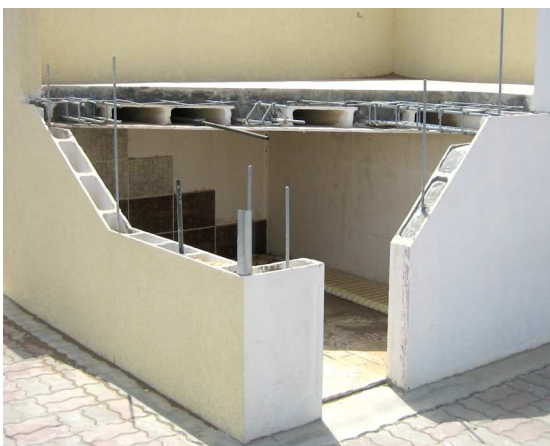
Display section showing Rapidfloor construction
