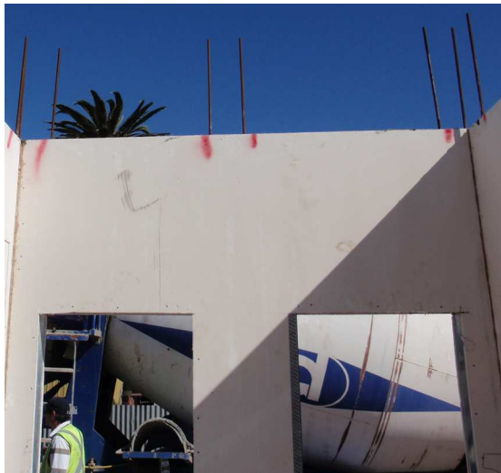
Reinforcement bars inserted ready for upper walls
