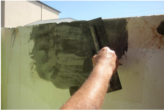
Repair to mid section of crushed panel
