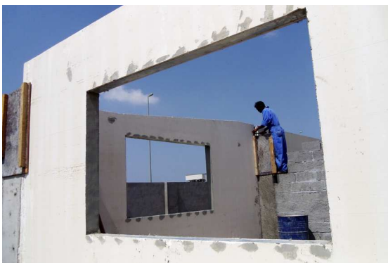
Vertical and Horizontal metal studs fitted in opening, screw heads flushed
